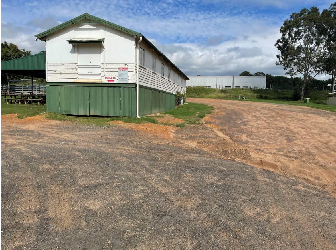
Figure 79 Heavy Vehicle Access road.
