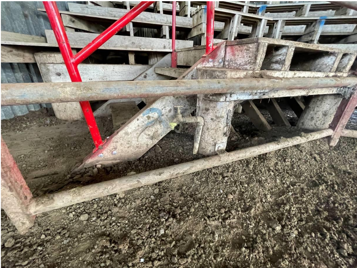
Figure 42 Tap in unsafe location, easily accessed by animals.
