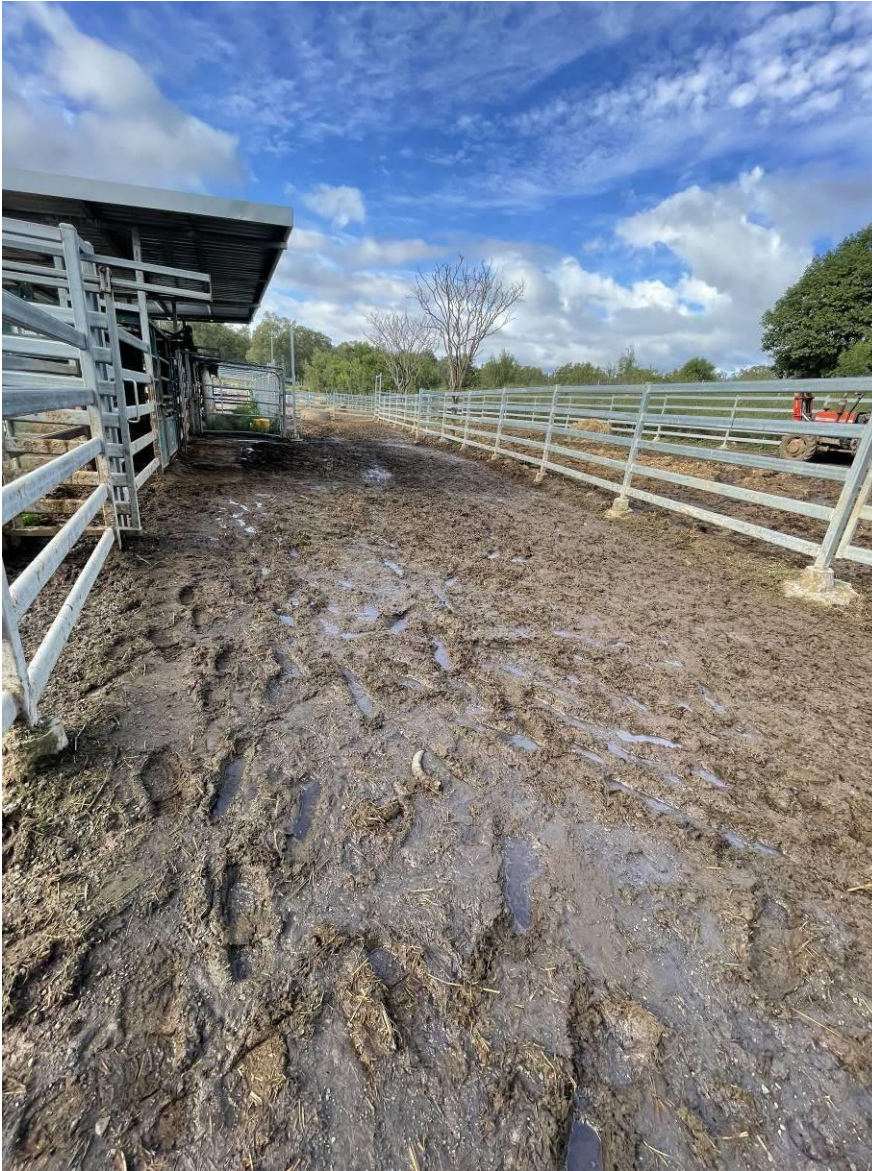
Figure 70 Yard beside vet crush - no drainage
