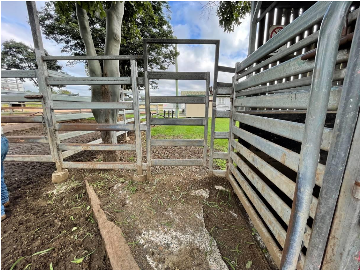
Figure 48 PA Gate in front of Animal Pound - pavilion entry/exit.
