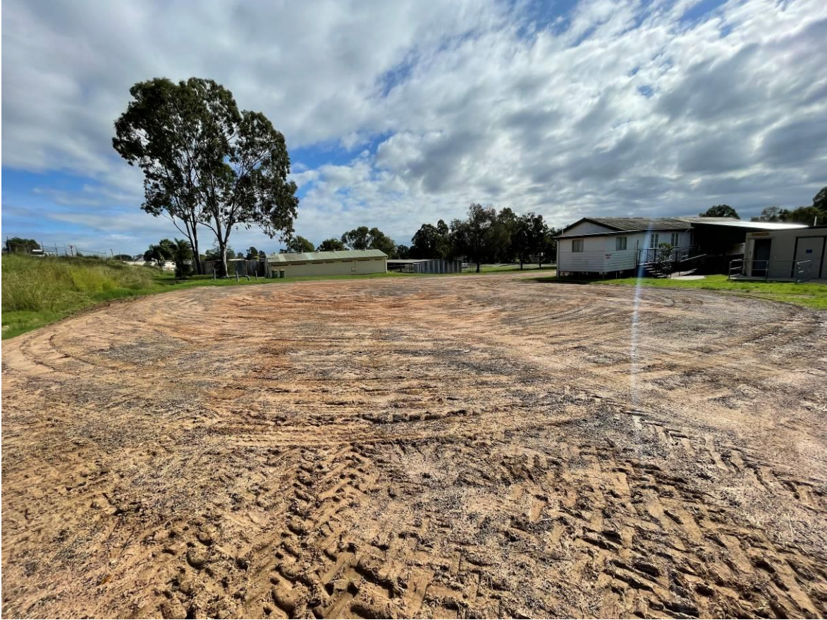
Figure 81 Surface is inadequate for heavy vehicles turning. No dust suppression.
