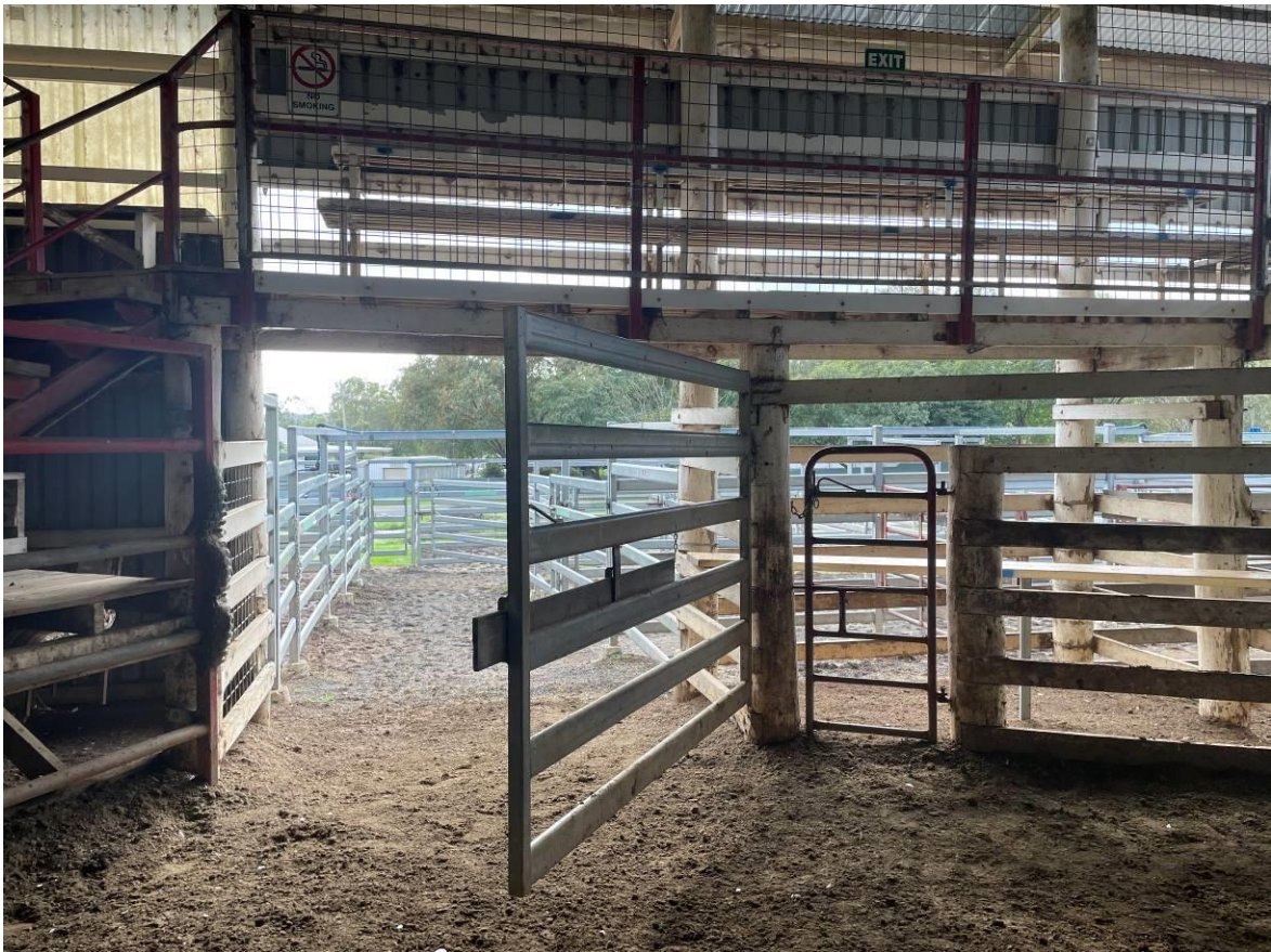
Figure 25 Not high enough for Ridden Horses to Exit – Height is 2.2m – 3m required.
