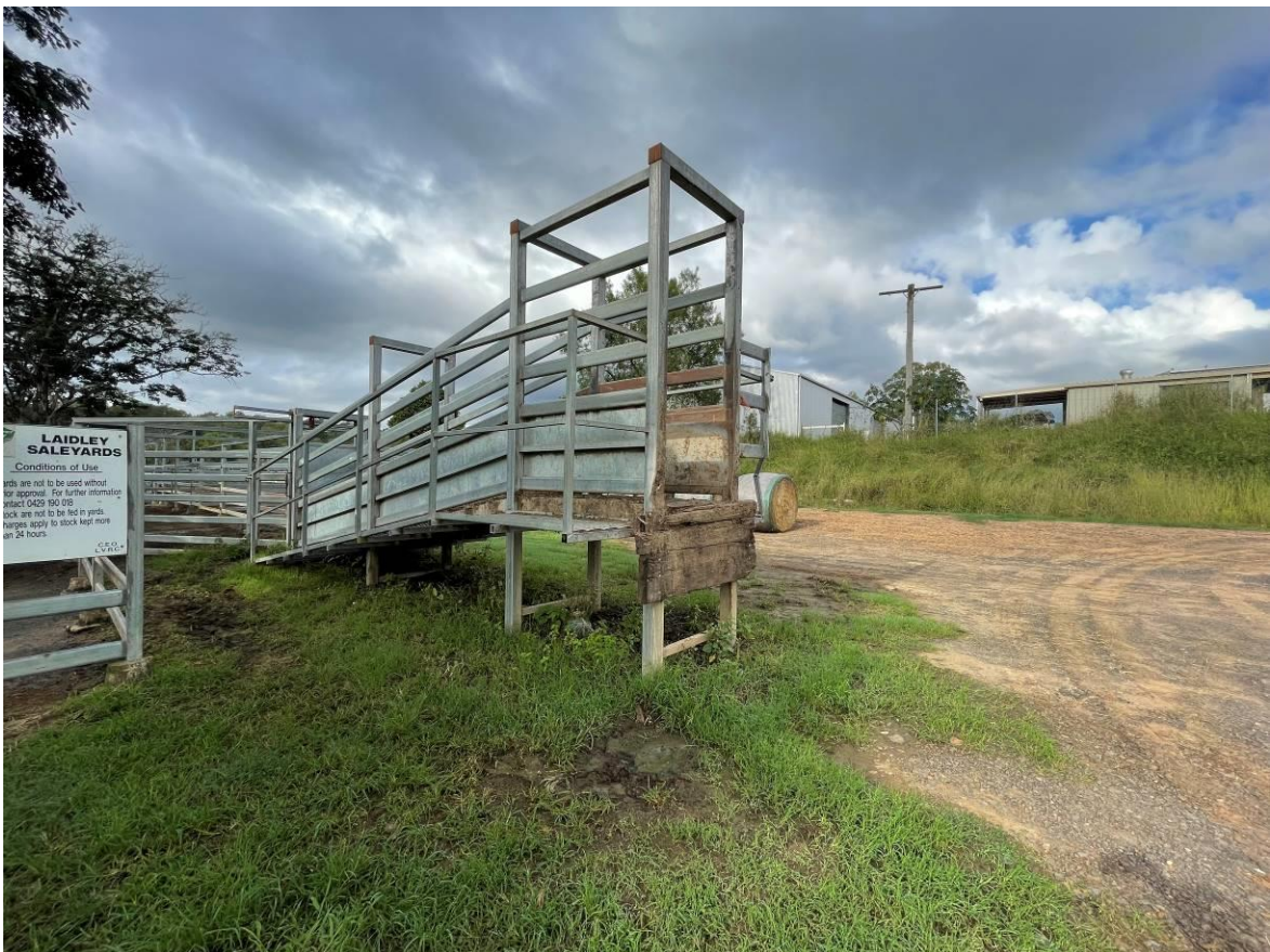
Figure 60 Second Loading Ramp (Southern Side) not compliant.
