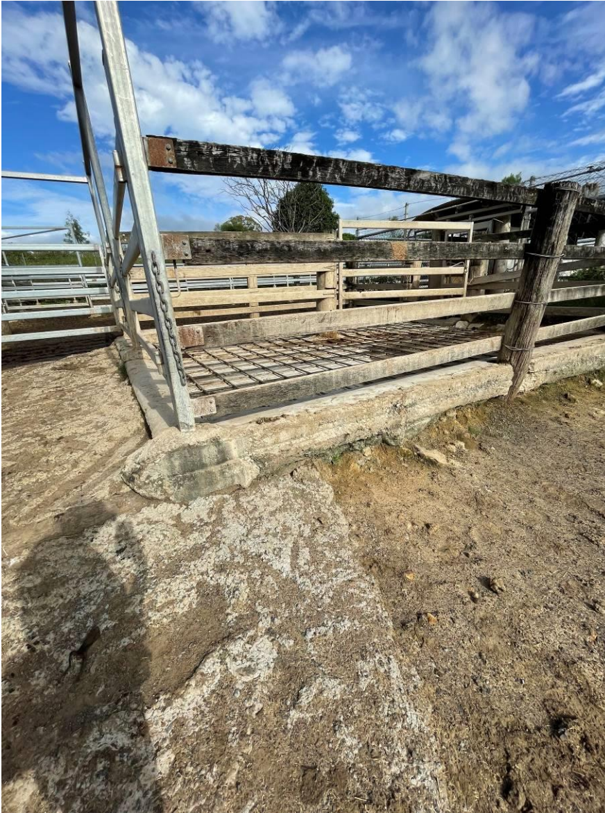
Figure 4 Dip Draining area. Runoff noted on the sides on the ramp and drainage pen. Green colouration is of concern.
