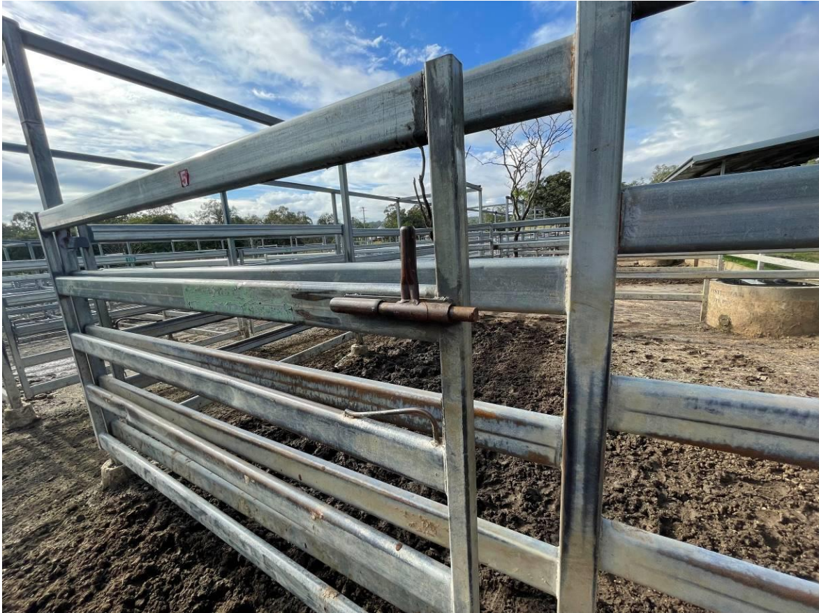
Figure 47 Gate not in correct position for cattle ramp loading and unloading safely - gate lock also upside down.
