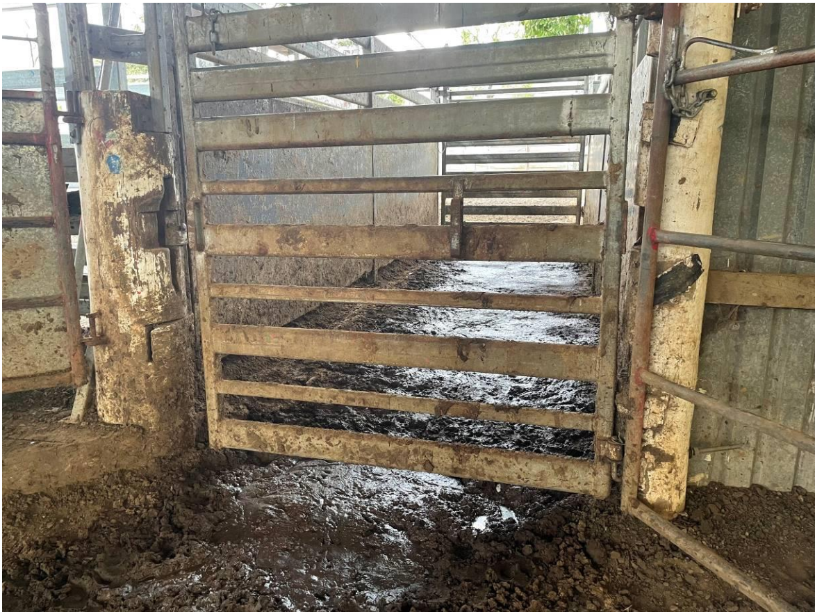
Figure 38 No stormwater controls in place in the Pavilion.
