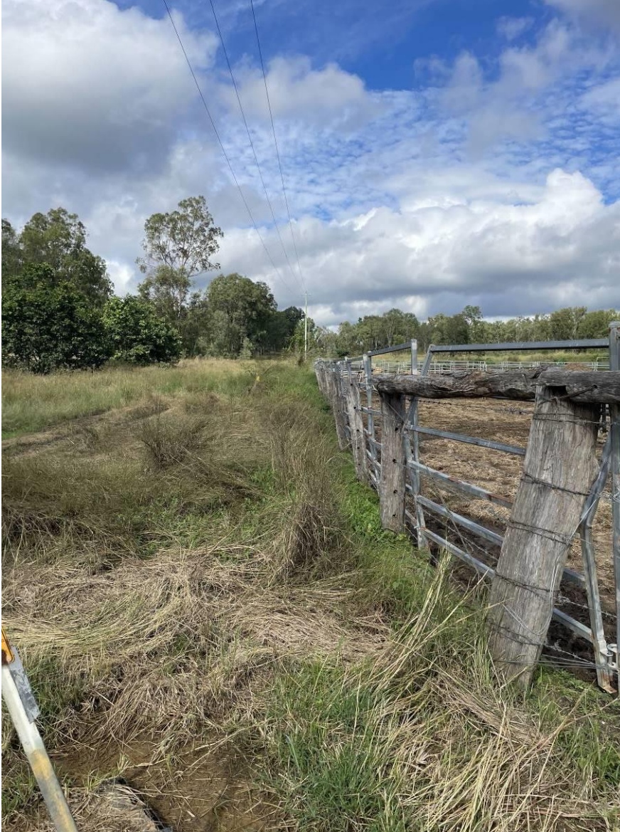
Figure 43 Temporary yard fence panels wired to old wooden posts.
