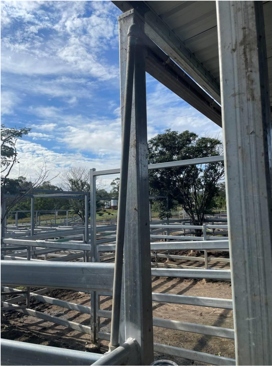
Figure 22 Water Transportation in Copper and PVC pipes
