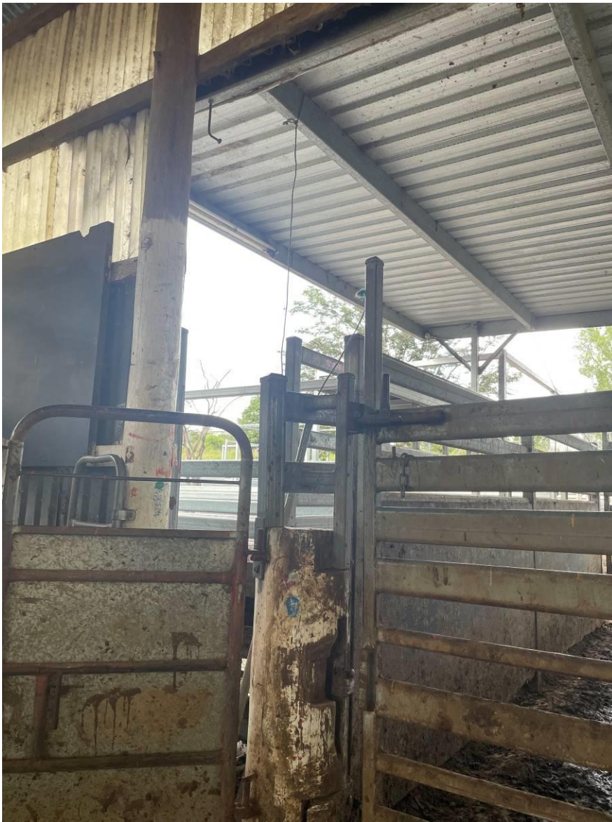
Figure 40 Gates in pound are pulled closed by a rope
