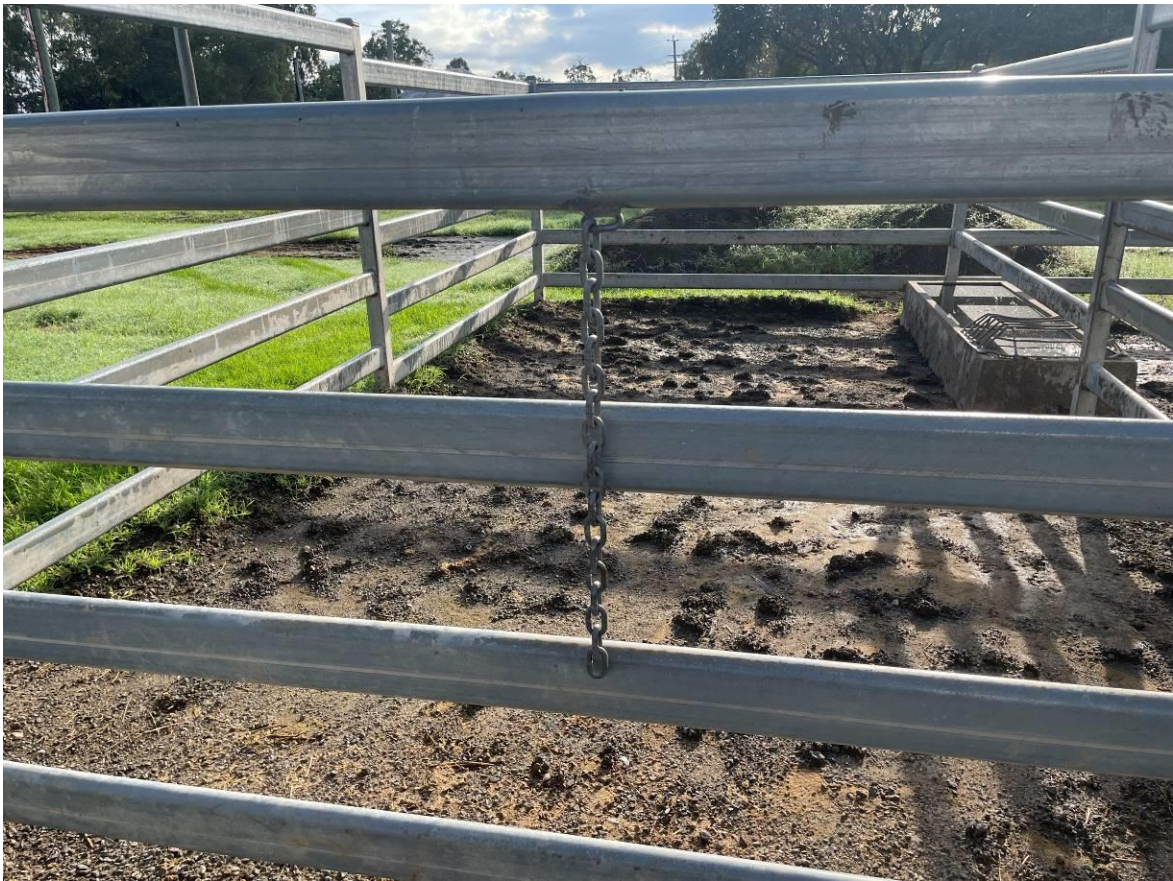
Figure 64 Chain for securing gates is too long. Needs to be no more than 200mm.
