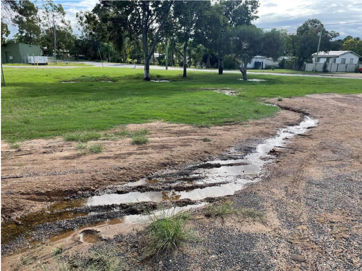
Figure 82 Drainage from Heavy Vehicle area is inadequate.
