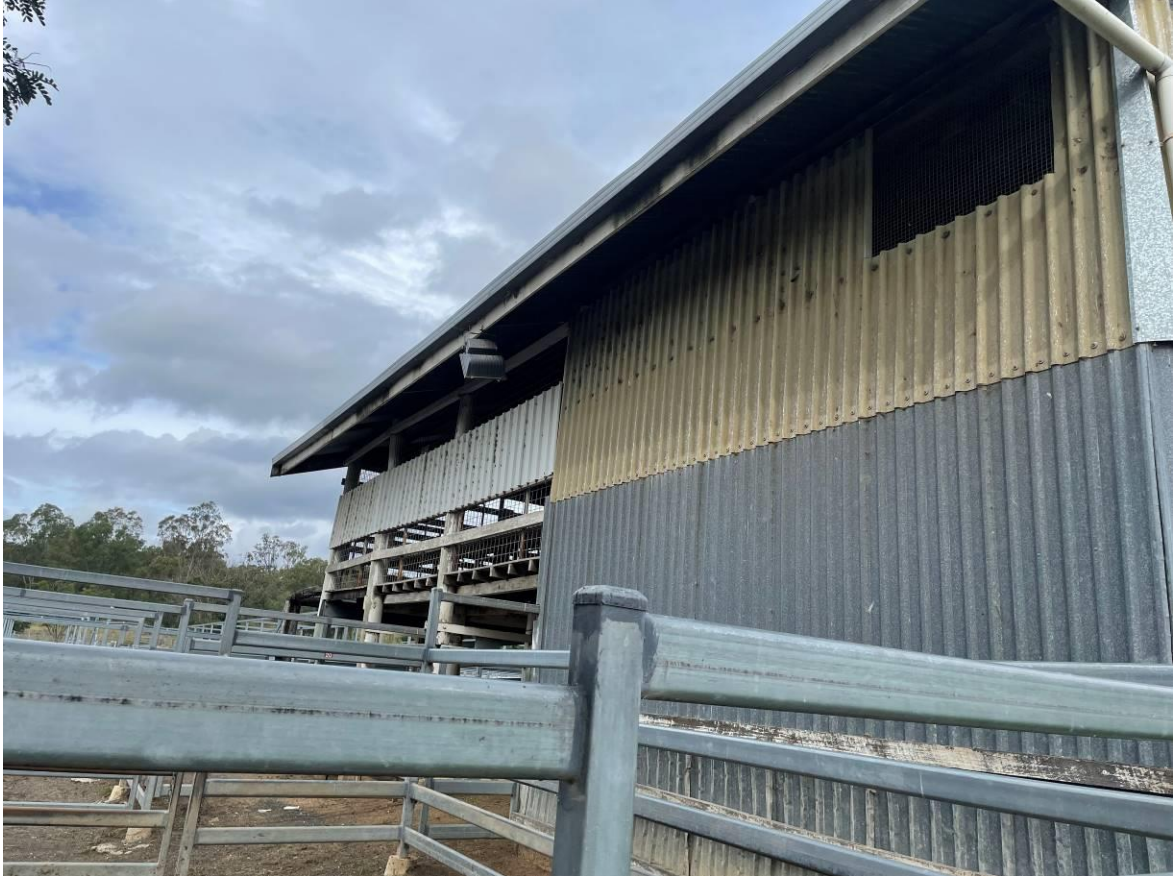
Figure 61 One Flood Light - Pointing East
