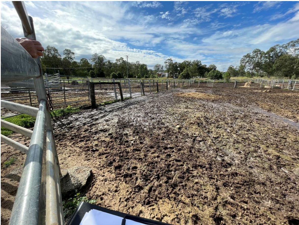
Figure 44 No stormwater or effluent controls in temporary yards.
