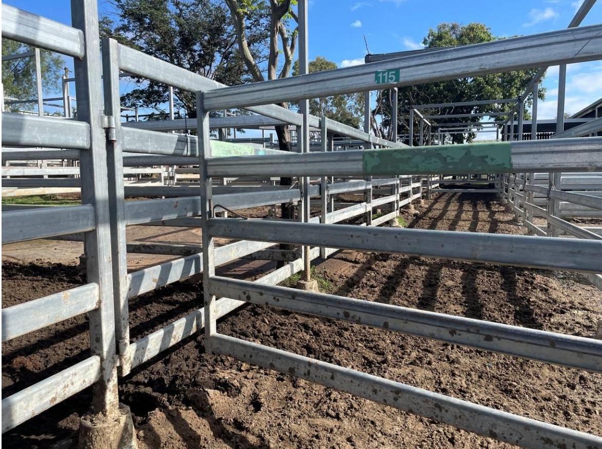
Figure 52 Laneway is correct width - 70-80 degree angle required.
