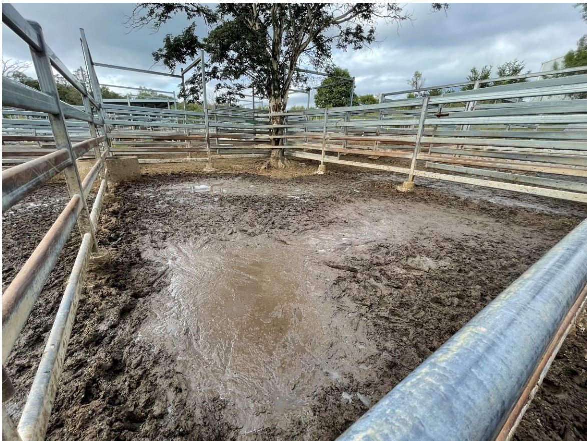
Figure 18 No adequate drainage - effluent does not drain away.
