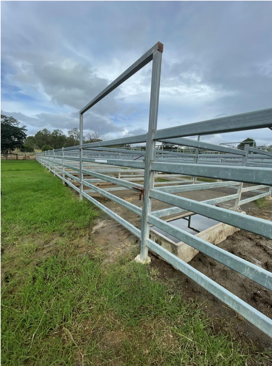
Figure 93 Exit gate on North side of yards - stock not secure.
