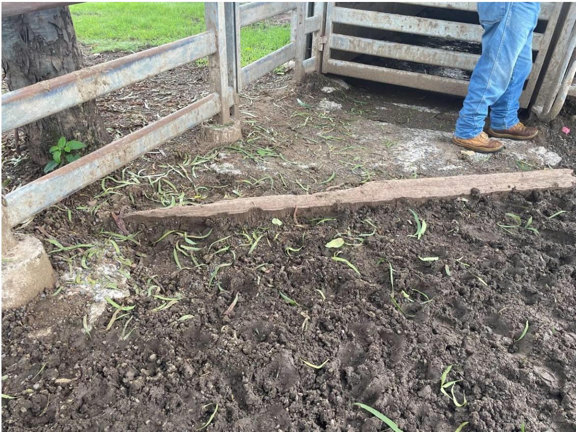
Figure 17 Yard Surface - Trip Hazard on Entry Point
