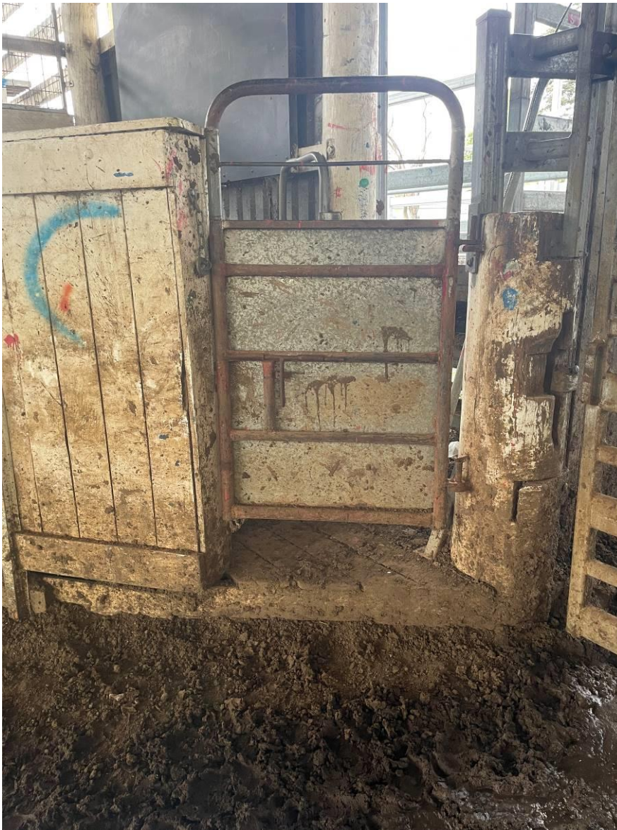
Figure 41 Not a slam shut gate. Bolt is located on the inside side of the gate in sale pen.
