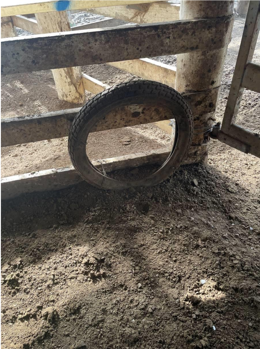
Figure 34 Tyre used to stop gate hitting fence inside the Pavilion
