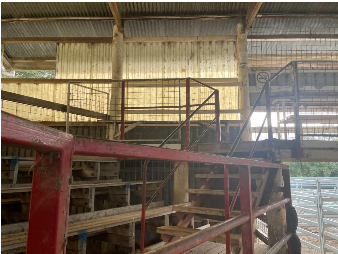
Figure 25 Not high enough for Ridden Horses to Exit – Height is 2.2m – 3m required.
