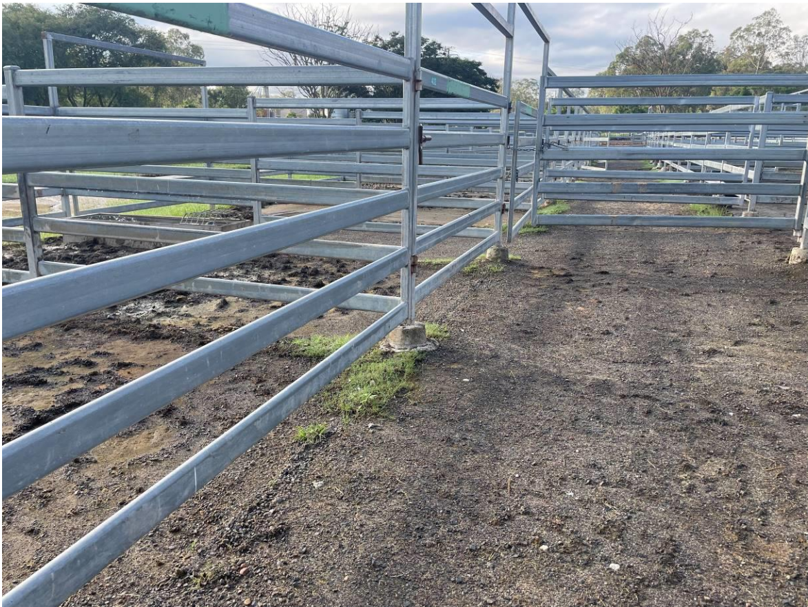
Figure 53 Laneways too wide - 3m gate swings freely open.
