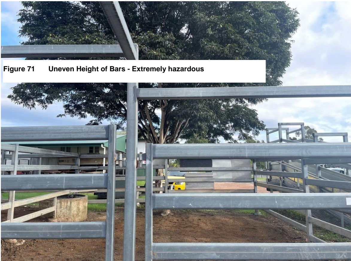
Figure 73 Gates tack welded to secure - uneven height on entry
