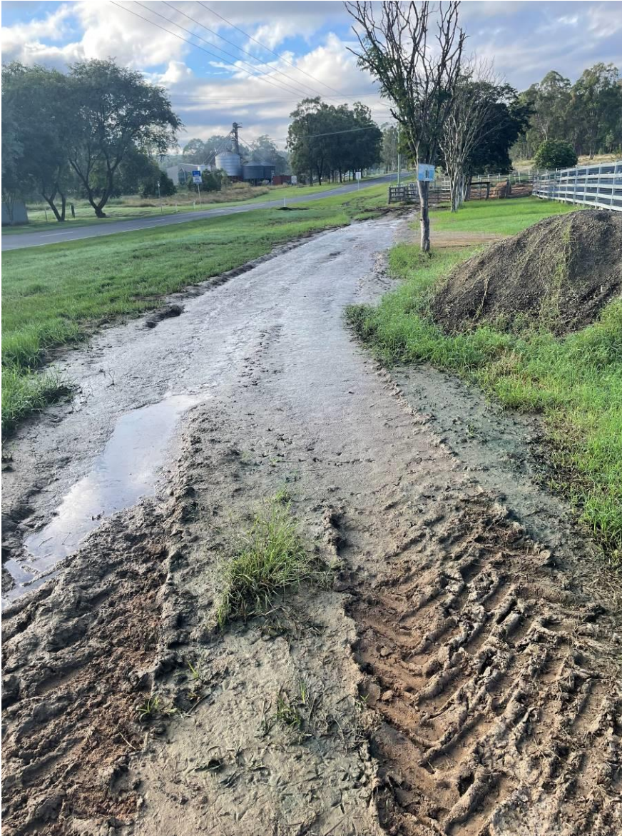
Figure 7 Stormwater/Effluent Flow from Yards into stormwater drain on the edge of the Laidley Rosewood Road.
